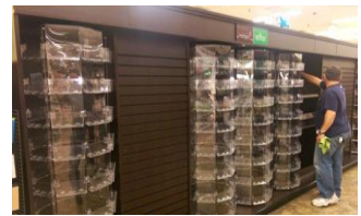
Store Fixture Install
