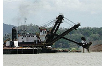
Bucket dredge working on the canal
